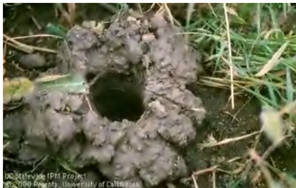
Figure 5. Holes dug by crayfish may cause unwanted seepage.
